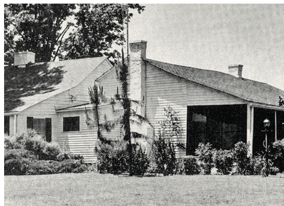
A partial view of the house at Loughborough, c. 1935.
