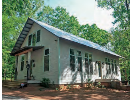
A photograph, c. 2011, of the Beaverdam Baptist Church after being moved to Athens, Georgia, and adapted for reuse as a residence.
